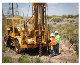
Subcontractors prepare to begin bore hole drilling in support of constructing a new Permanent Ventilation System at WIPP.
